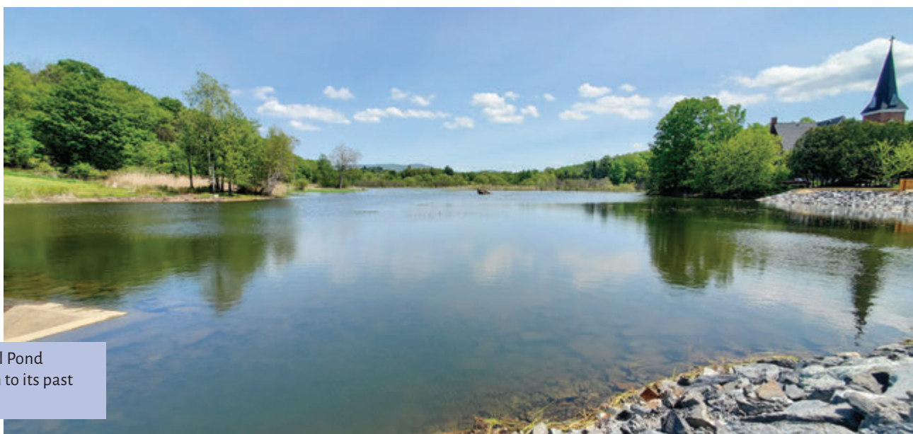
View of the front of the dam.
